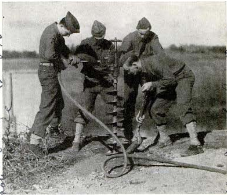
Pneumatic auger speeds setting of dynamite charges by demolition squad
